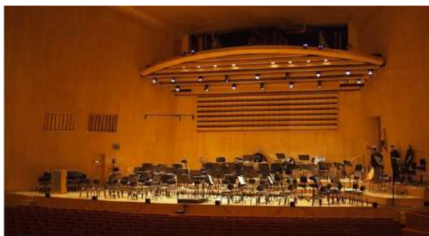
Figure 2. Photo showing new sound translucent stage canopy and the organ chamber opening at the back of the canopy (Photo by Alf Berntson, Artifon [7]) Photographs and figures show the design of the concert hall organ prior to the installation of the concert hall organ including a new canopy.
